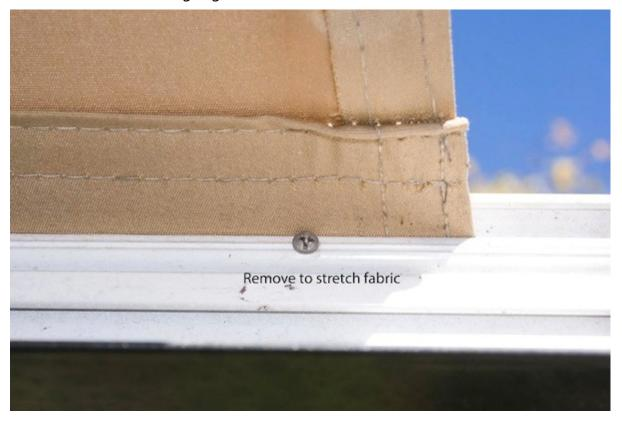
Check the outward extension limit. Because the fabric has stretched there is probably no tension on it at full extension. Check at the 'elbows' of the arms. You should have enough gap there to see both cables. If not turn the extension screw, hole farthest from MH, CCW with 4 mm allen. Figure 3.
